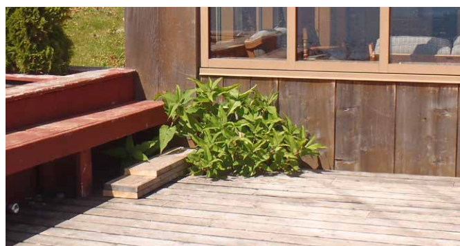
Knotweed is able to grow through decks and building foundations as this photo showing Himalayan knotweed demonstrates.
